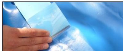
. Pose the adhesive tape on the damaged zone.
